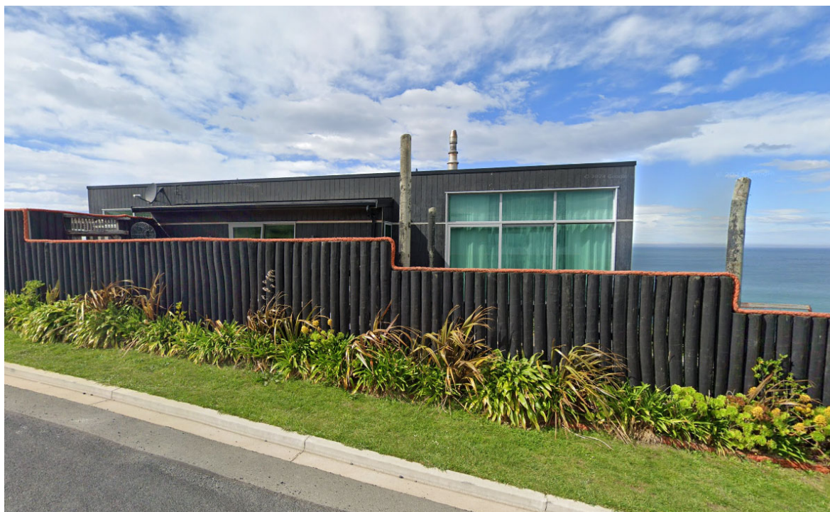
Figure 1: View of property looking southeast
