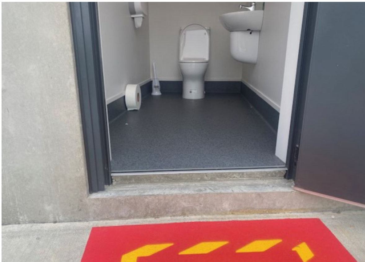
Figure 1: As-built single external step to toilet facility
