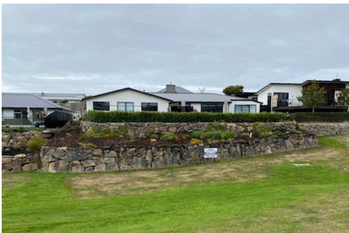
Figure 1: The retaining walls
