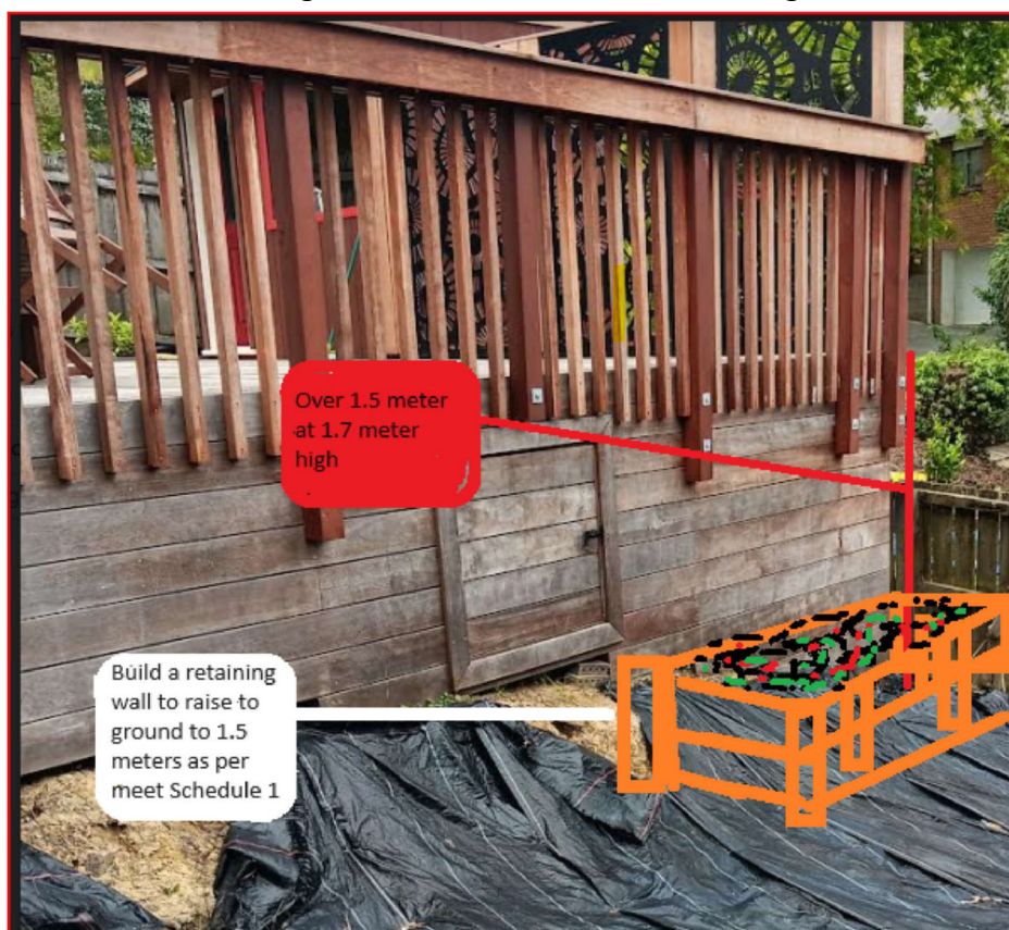
Figure 1. Building surveyor's annotated photo showing maximum height of deck
