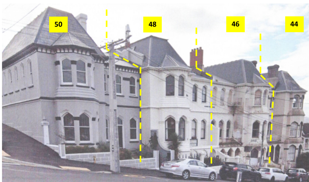
Figure 1. View of 50, 48, 46 and 44 Manor Place from the street
