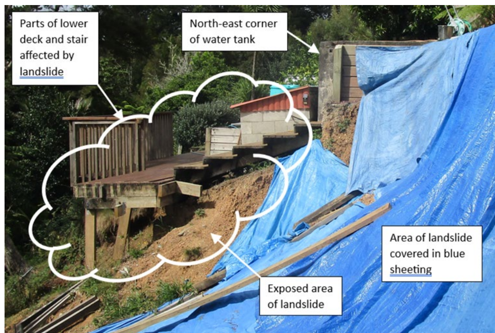
Figure 5. Lower deck, access stair and water tank 13
