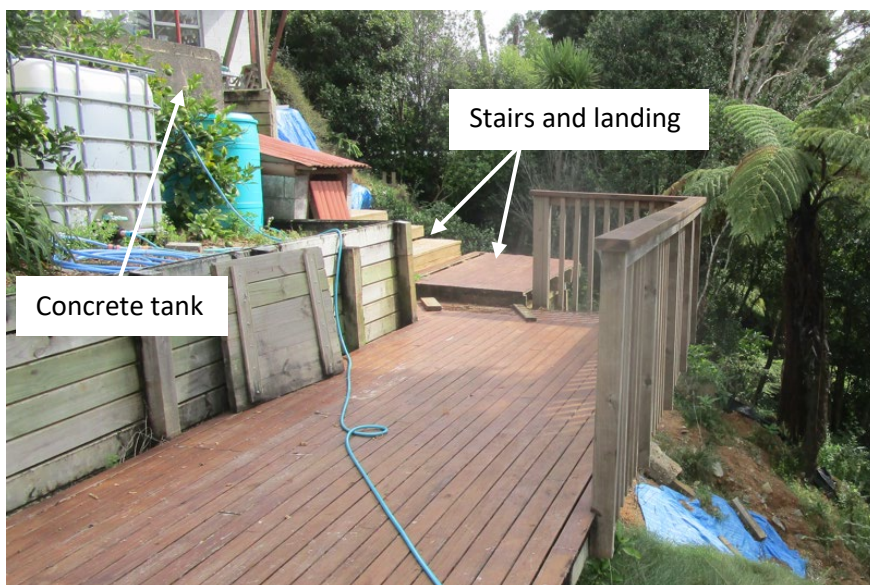
Figure 3. View of lower deck and landing
