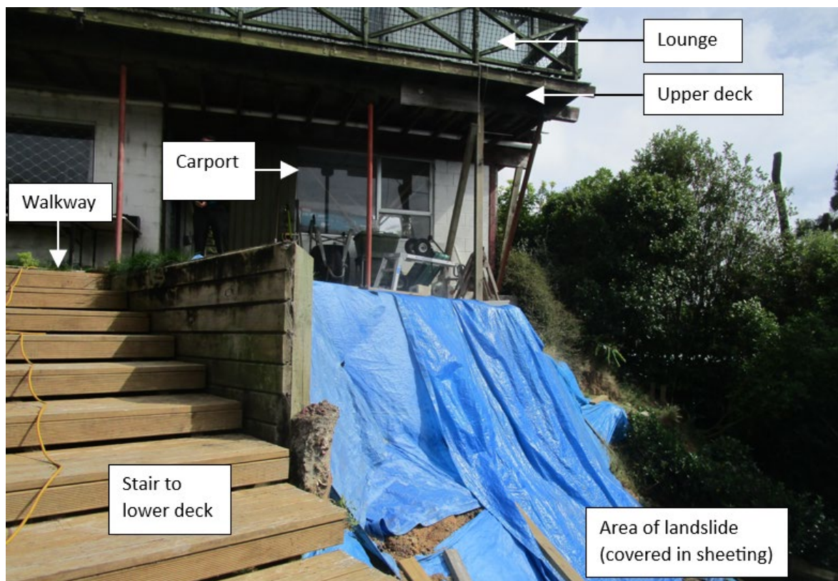
Figure 1. Part of landslide on the east side of the dwelling
