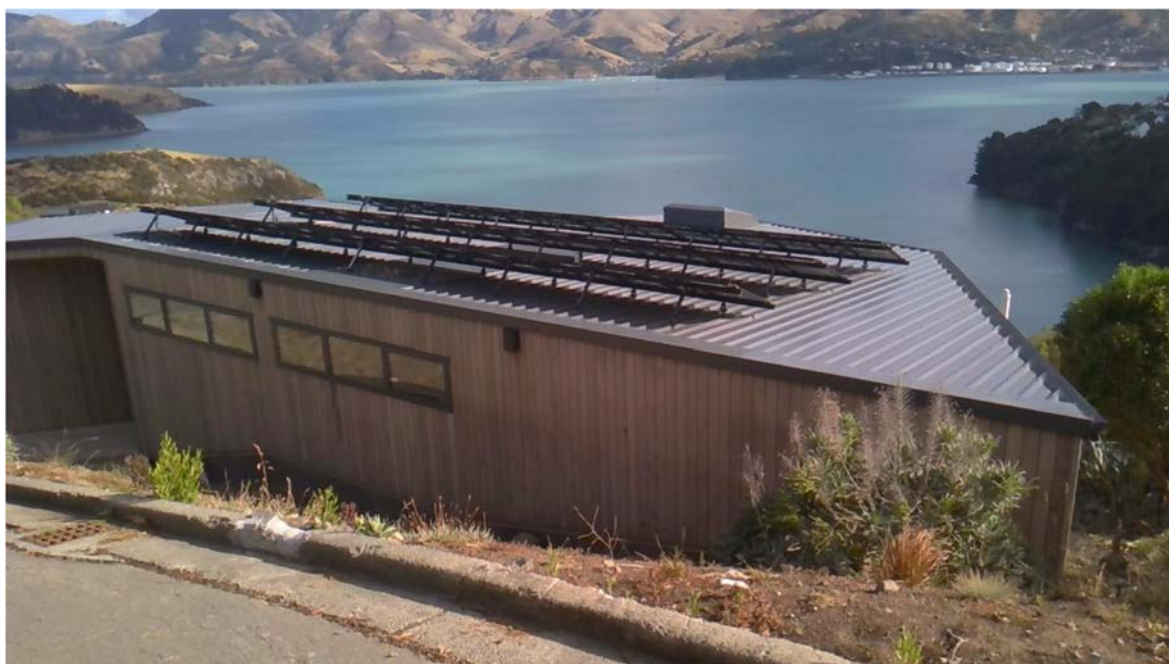
Figure 1: Rear elevation of dwelling looking northwest 1
