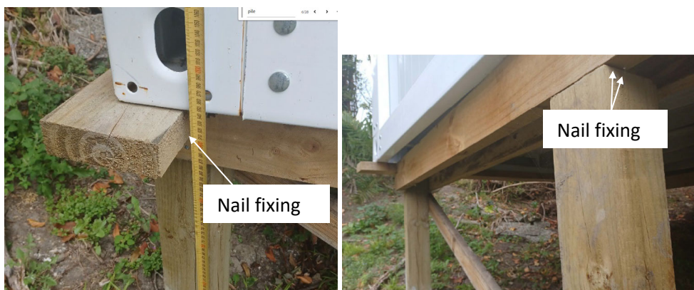
Figures 2 & 3: showing pile and bearer connections
