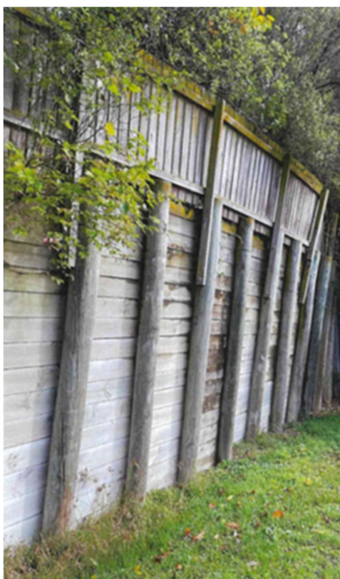
Figure 1: The retaining wall under consideration
