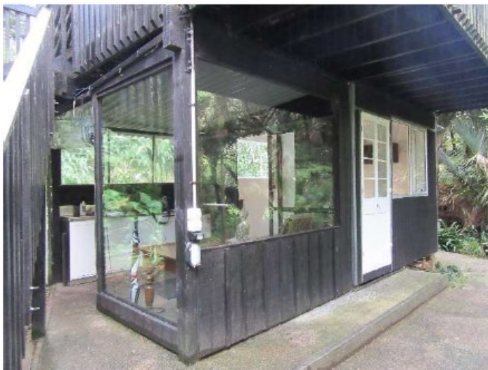
Figure 2: Photograph showing partially enclosed area on ground level.
