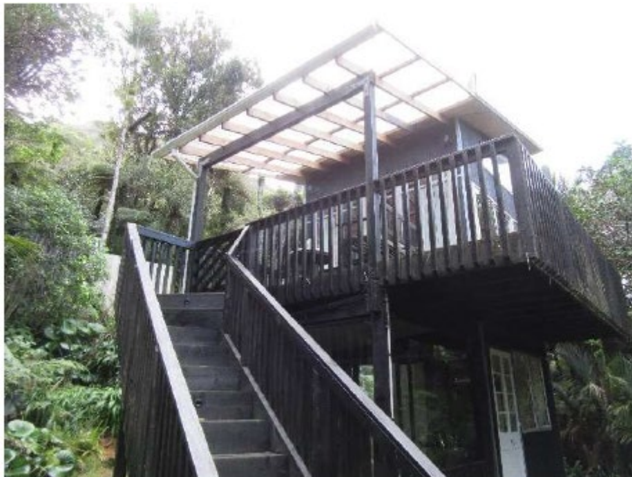
Figure 1: The building under consideration.
