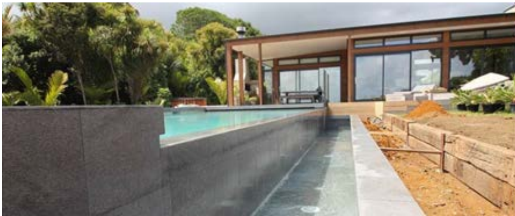
Figure 1: The pool's infinity edge and balance tank during construction
