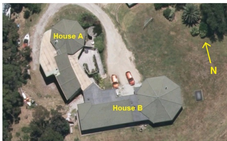
Figure 2: Aerial view of Houses A and B
