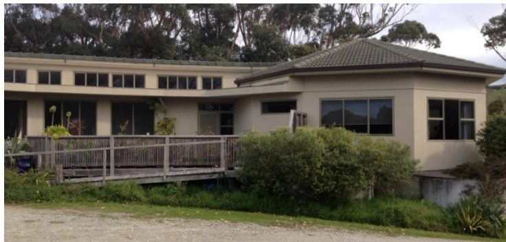
Figure 1: East elevation of House A
