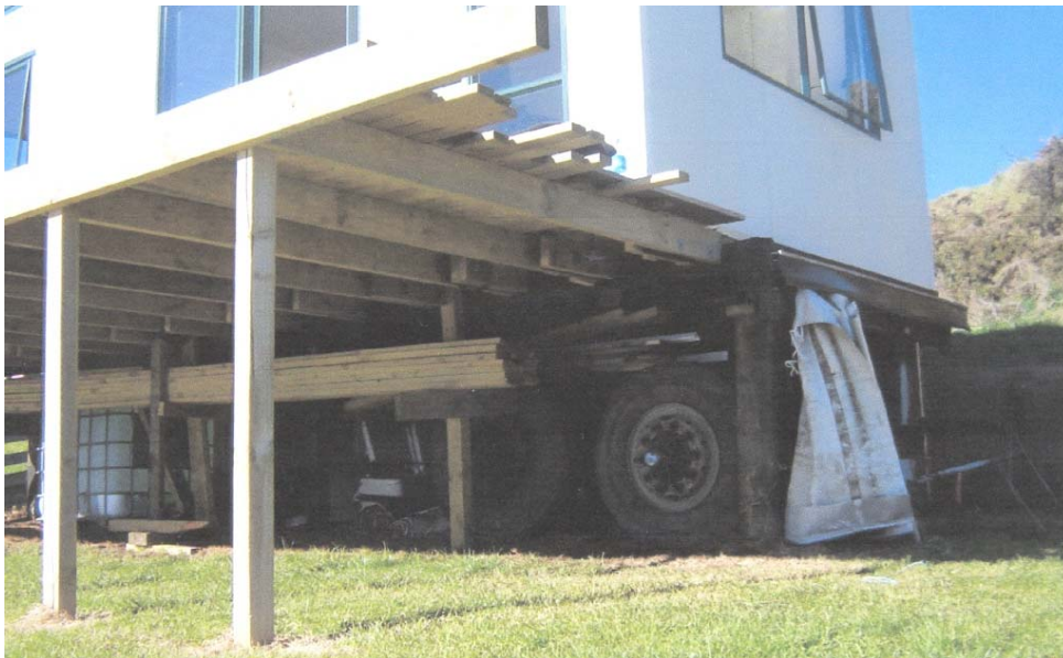
Photograph 2: The axles and wheels remain in place
