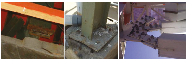
Figure 21: Weld failure of rafter attachment to concrete support (left); Base plate deformation (centre); Steel bracing cleat fracture (right)
