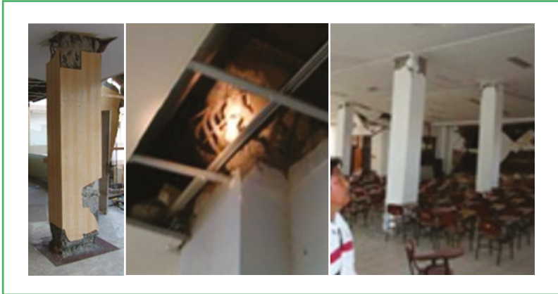
Figure 15: Column hinging top and bottom (left); Top of column hinging failure above suspended ceiling (centre); Columns out of plumb (right)
