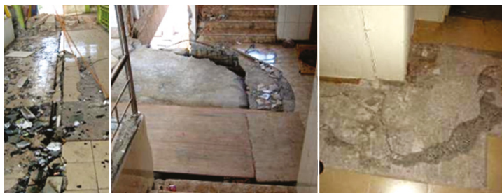
Figure 18: Structural movement joint in suspended slab (left); Floor diaphragm damage (centre); Punching shear failure in suspended slab at end of shear wall (right)
