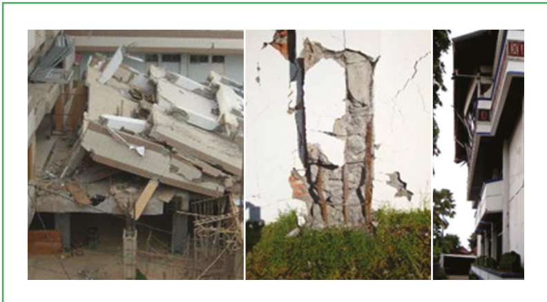
Figure 16: Weak column-strong beam frame collapse (left); Column flexural hinging with concrete crushing and reinforcing steel fracture (centre); Falling hazard from partially detached wall cladding panel (right)
