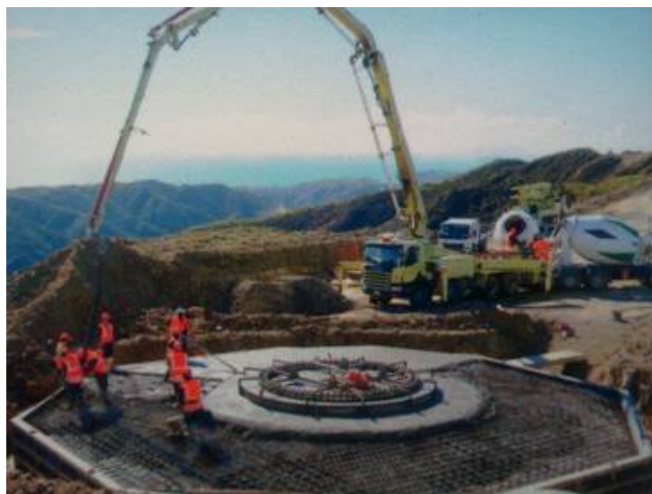
Photos 2-3: Completed turbine and base under construction
