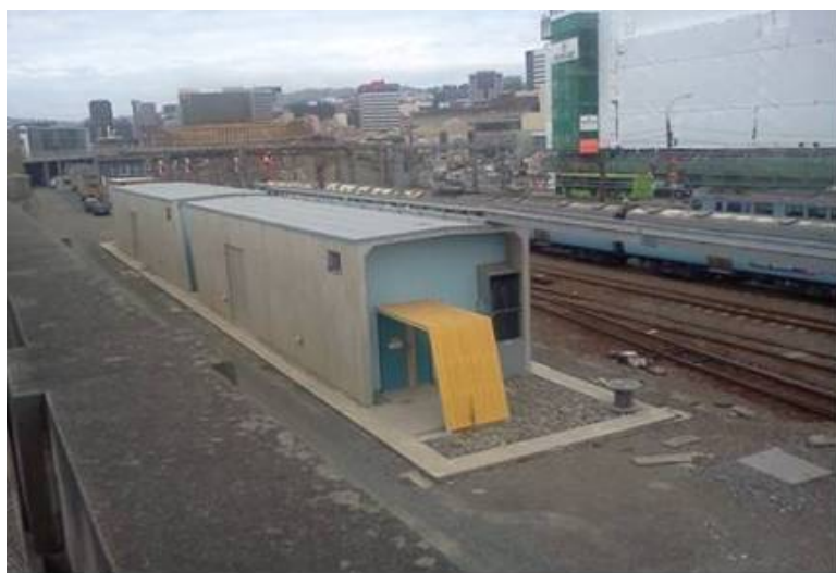
Photo 4: Rail network substation
