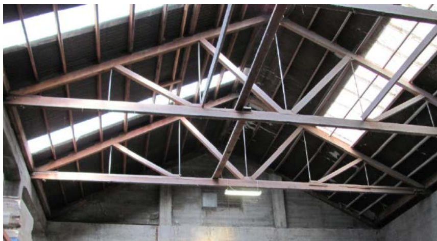
Figure C2E.1: Example of a flexible diaphragm
