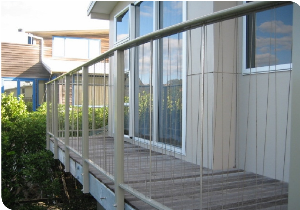
Figure 4.13 Sloping wires changing direction within the rails
