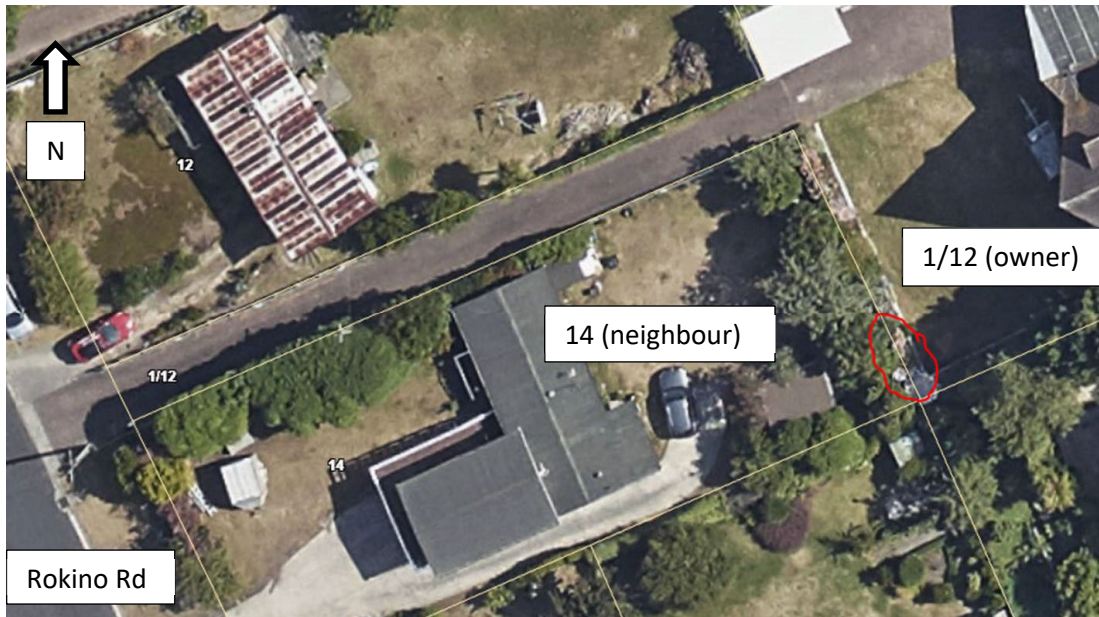
Figure 1: Aerial photograph provided by the authority, showing the approximate location of the new section of punga wall, circled in red
