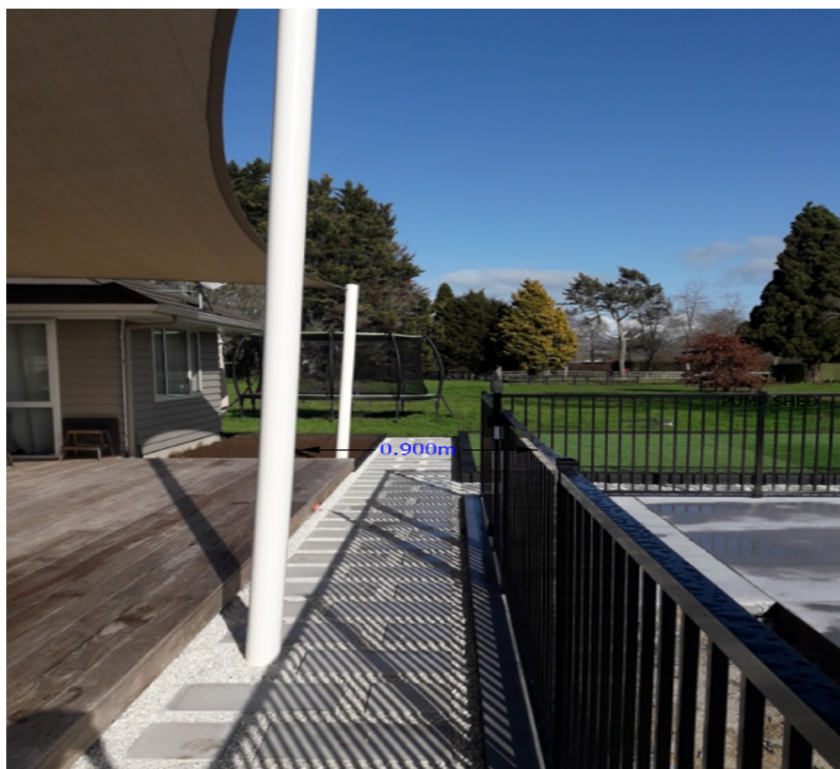
Figure 1: The shade sail pole and the pool barrier
