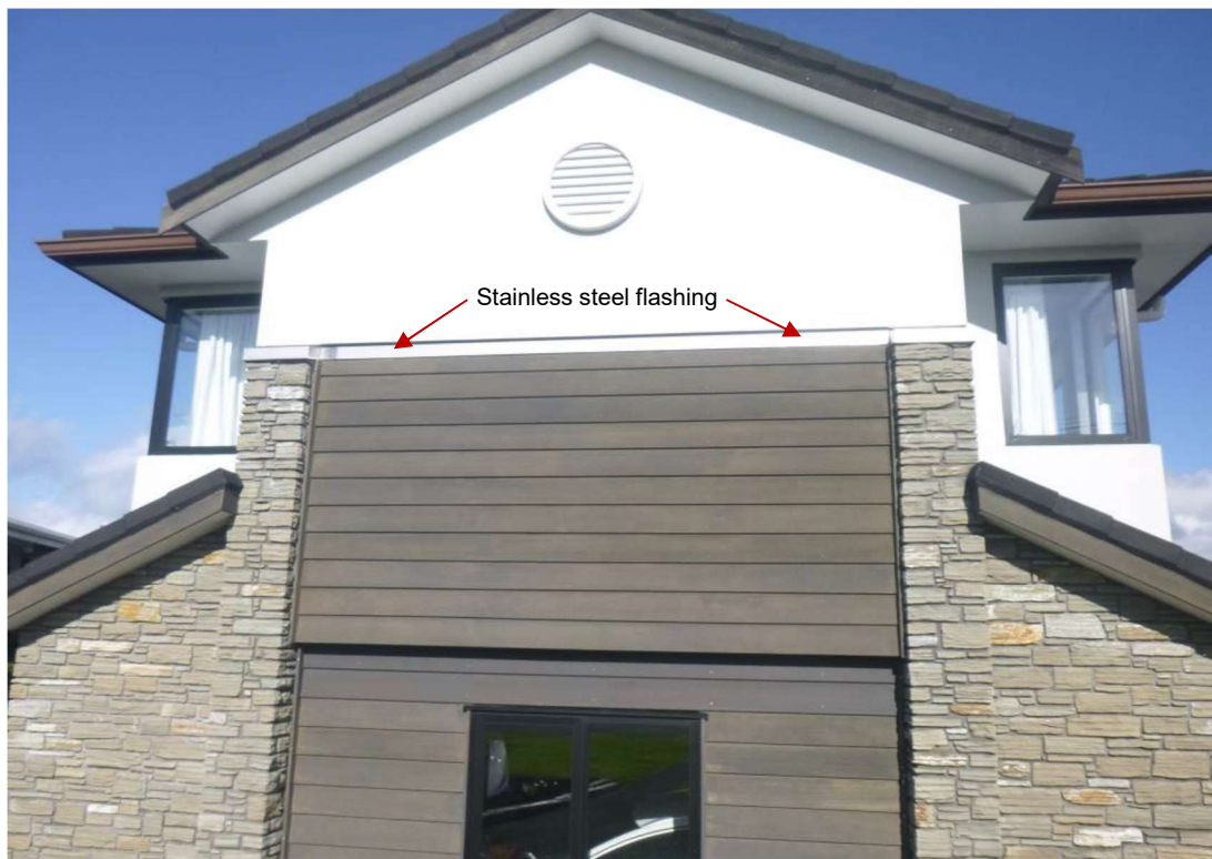
Photo 4: Stainless steel flashing, north elevation gable wall
