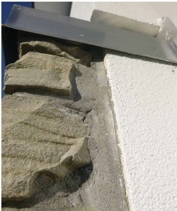
Photo 3: Stone schist cladding to EIFS cladding junction, northwest corner
