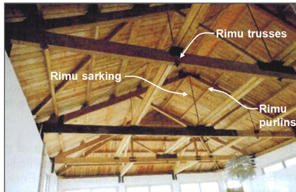
Figure 1: Original roofing timbers
