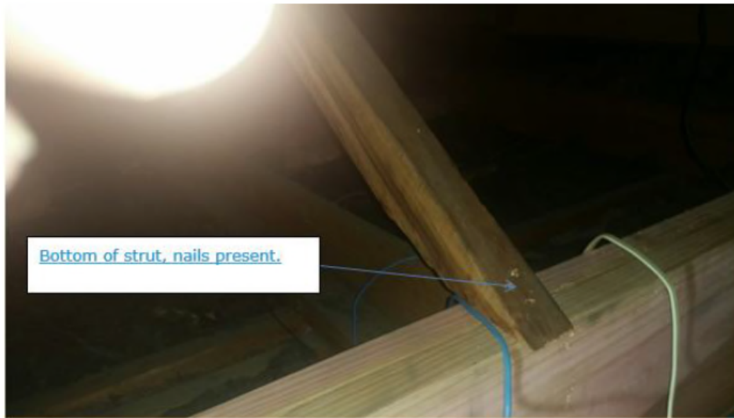
Photo 2. Bottom of strut with very little splitting of the timber.
