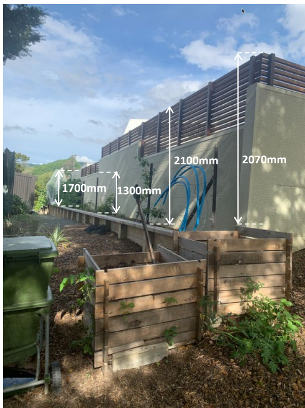
Figure 5: The boundary fence viewed from the neighbouring property, looking east
