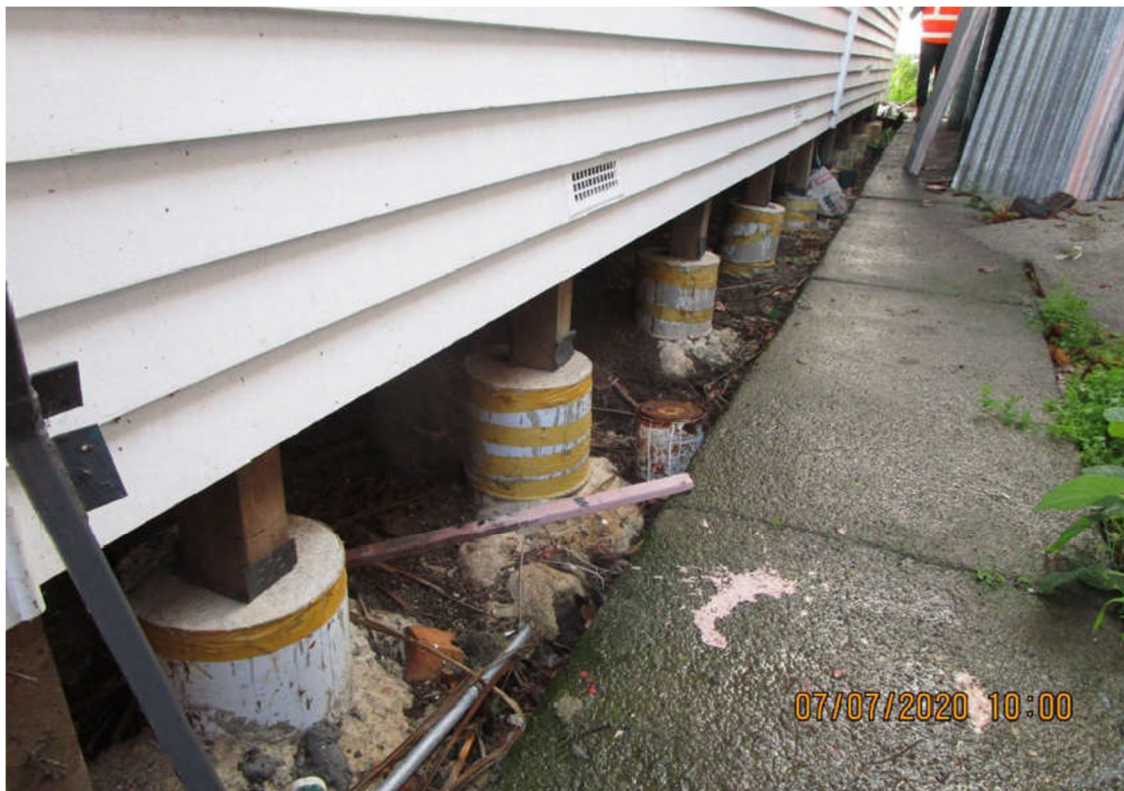
Figure 1: Concrete piles on the south side of the property
