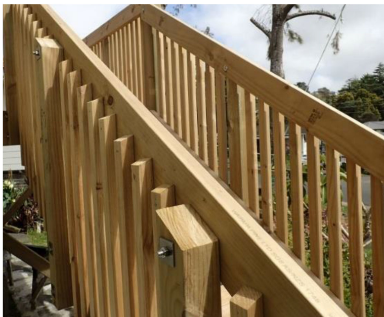
Figure 1: The stair handrails 1
