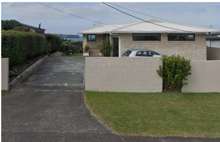
Figure 1: View of dwelling from road, looking east 1
