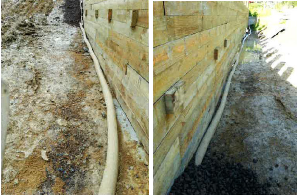
(a) View looking northwards
