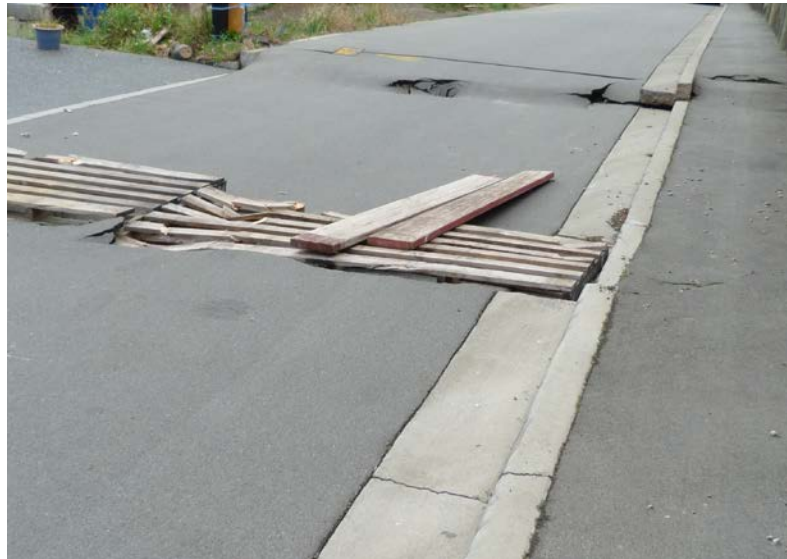
Figure 3: Graben formed in extension area of a mass movement feature (A graben is a depressed block of land bordered by parallel defects)
