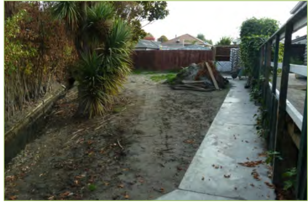
Liquefaction ejecta alongside culvert
