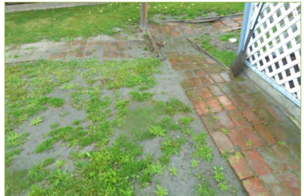
Undulations in lawn, liquefaction ejecta removed
