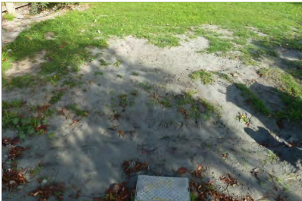
Liquefaction ejecta on lawn
