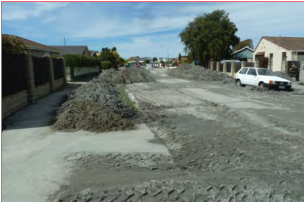
Liquefaction ejecta piles along Androssan Street
