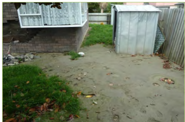
Liquefaction ejecta and brickwork damage
