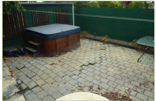
Undulations in paving area
