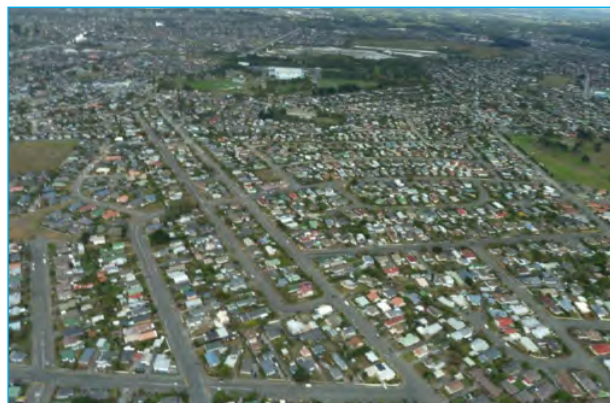
Aerial photo of North New Brighton showing little damage
