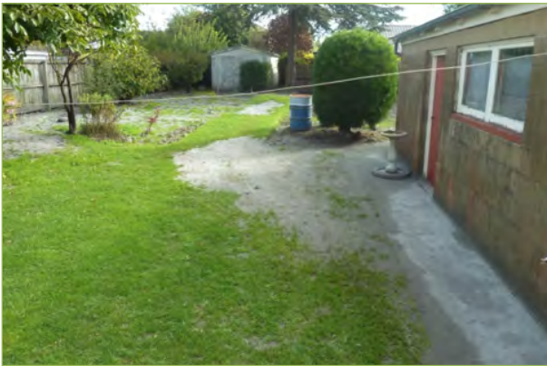
Liquefaction ejecta in many places on lawn
