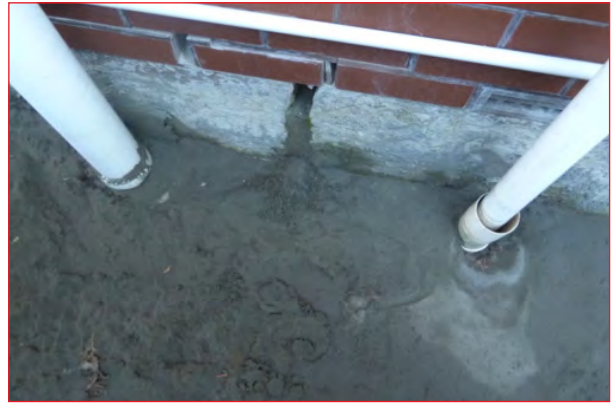
Foundation damage
