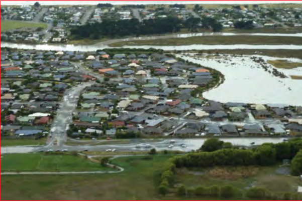
Aerial photo showing liquefaction ejecta on Seabreeze Close
