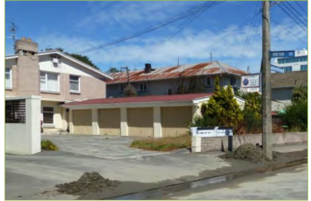
Piles of sand along the footpath
