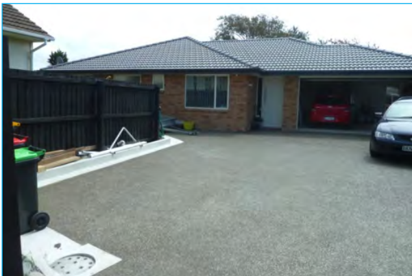
Undamaged concrete driveway and kerbing
