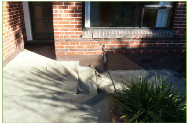
Foundation damage
