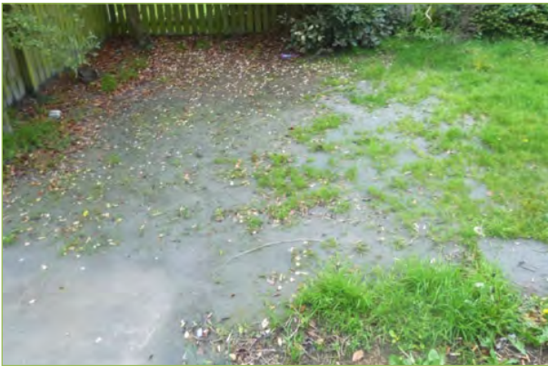
Liquefaction ejecta on lawn
