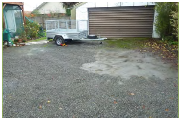
Isolated area of liquefaction ejecta
