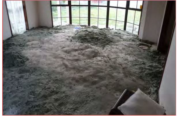
Liquefaction ejecta inside house
