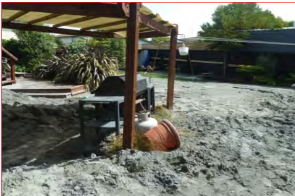
Liquefaction ejecta around property
