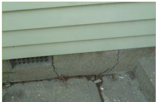
Foundation damage
