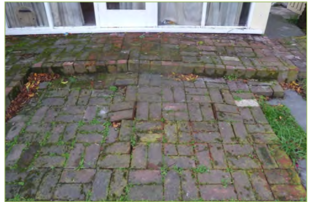
Undulating paving bricks
