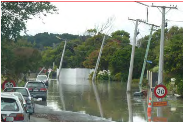
Flooding and lateral spreading damage to power lines
