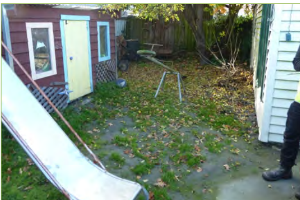
Liquefaction ejecta on lawn
