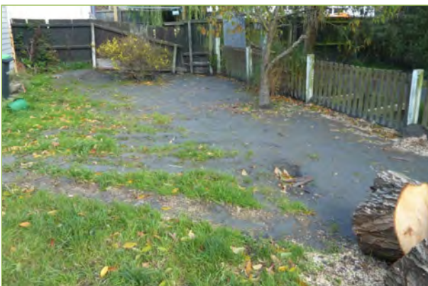
Liquefaction ejecta on lawn
