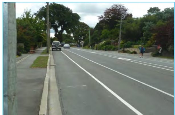
View of Centaurus Road with little damage
