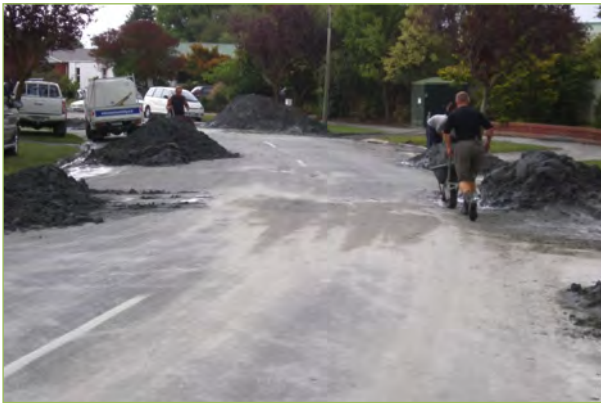
Liquefaction ejecta in piles on road
