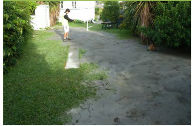
Liquefaction ejecta on lawn
