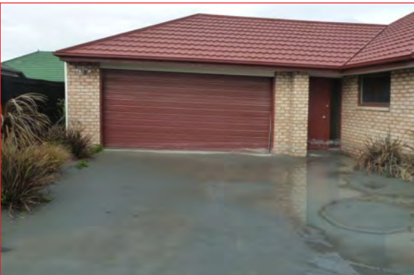
Large amounts of liquefaction ejecta and tilting dwelling
