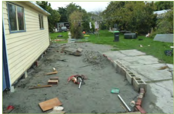
Large area of liquefaction ejecta on lawn
