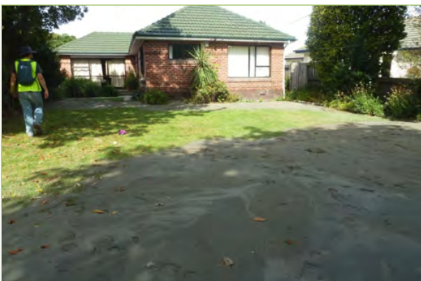
Liquefaction ejecta, dwelling tilting
