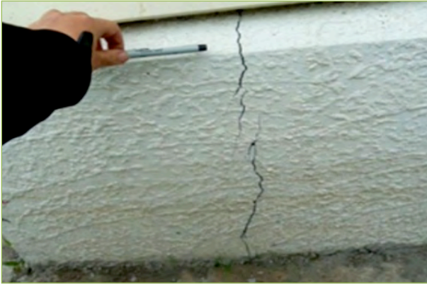
Foundation damage
