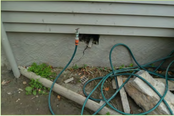
Foundation damage
