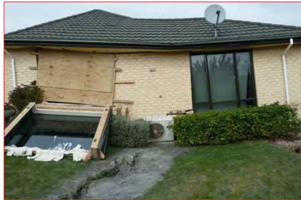
House deformed by lateral spreading
