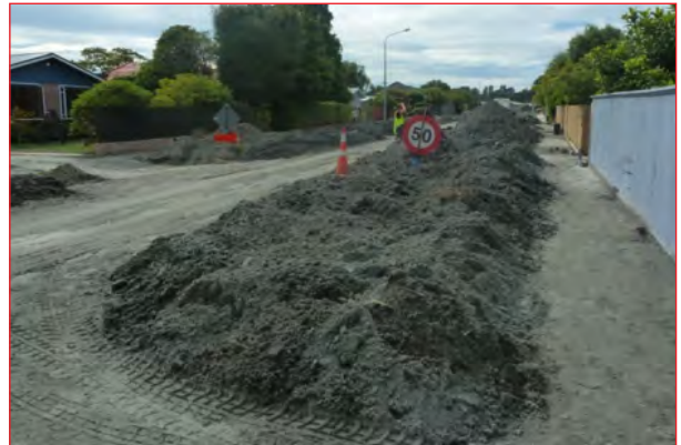
Liquefaction ejecta piles along Avonside Drive
