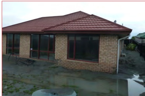
Large amounts of liquefaction ejecta around property
