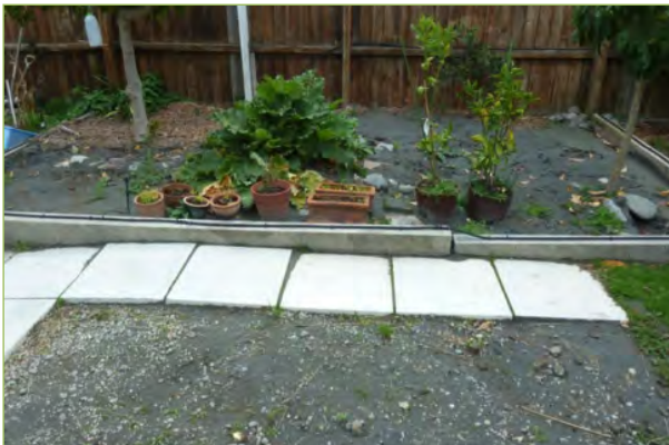
Liquefaction ejecta in planter with undulating pavers
