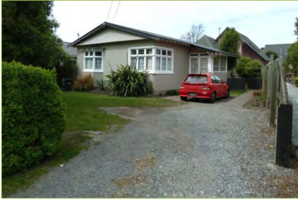
Undulating lawns and liquefaction ejecta
