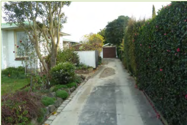
Cracking and ejected sand on driveway
