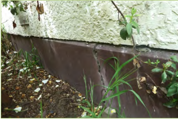
Foundation damage
