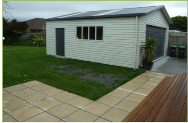
Liquefaction ejecta on lawn
